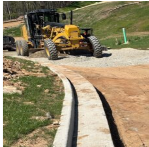
Subbase prep. at 1B
