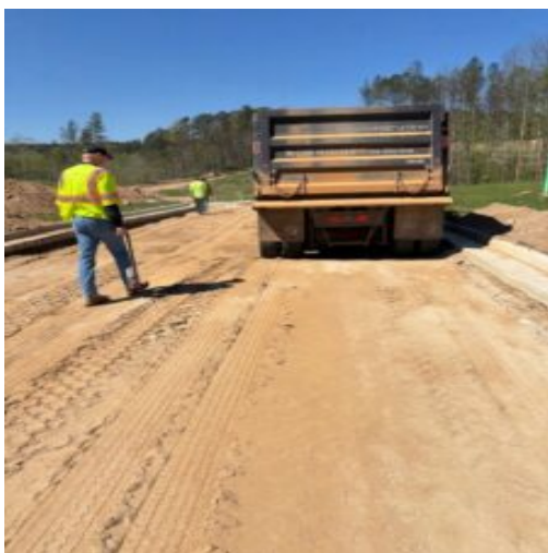
Subgrade proof roll at 1B
