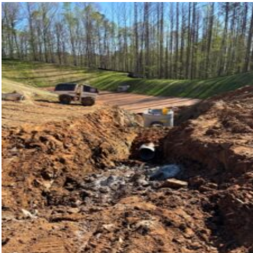
Trench rock at C line
