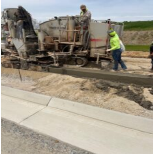
Installing type 7 curbing at Nature Walk
