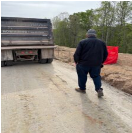
Proof rolling subbase stone at Nature Walk for curb installation
