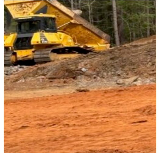
Placing rockfill at unit 4 phase 3
