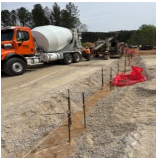
Installing type 7 curbing at Nature Walk
