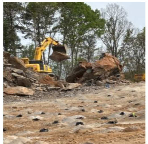
Breaking and hauling blast rock
