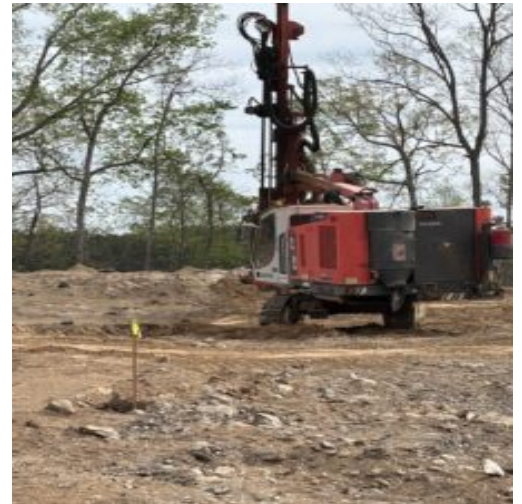
Drilling rock at cul de sac phase 2
