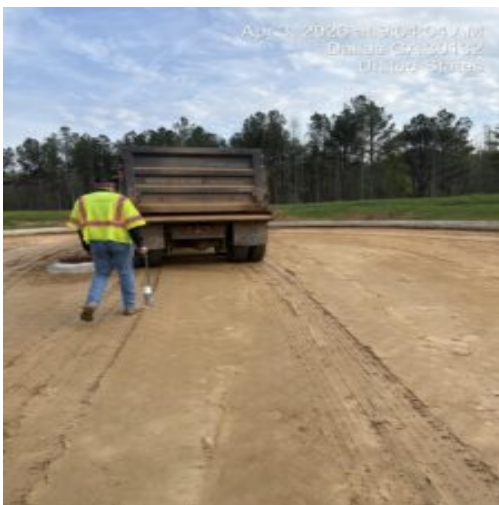
proof rolling with loaded truck
