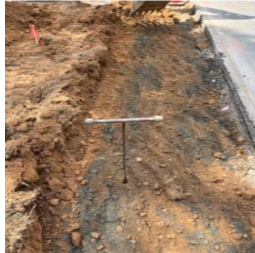
Observing subgrade for new curbing at round about
