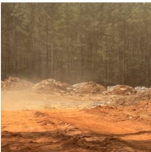
Excavated stockpiled rockfill at unit4 phase3
