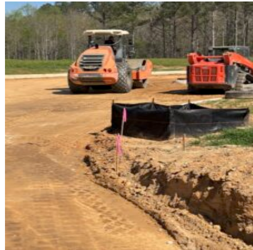
Compacting subgrade at phase 1A
