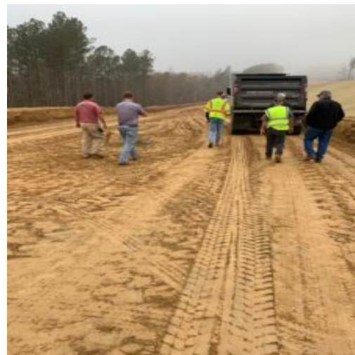
Proof roll observed by county, paving and grading contractors
