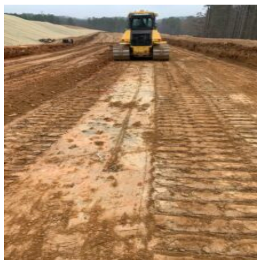
Repair area clipped using dozer
