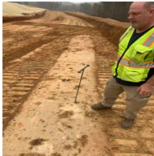
Repair area clipped using dozer
