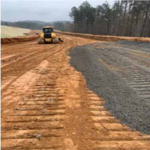
Placing base stone after clipping sub grade
