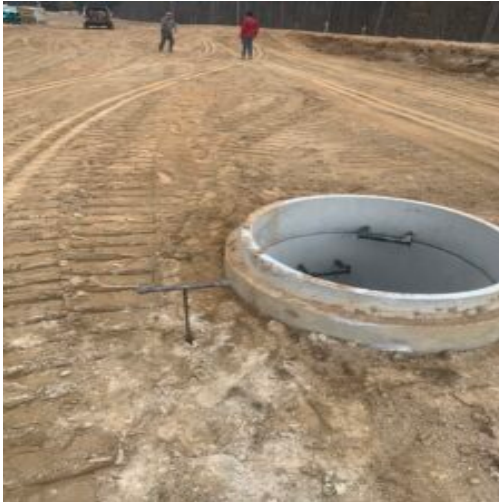
Loose compacted areas around manholes
