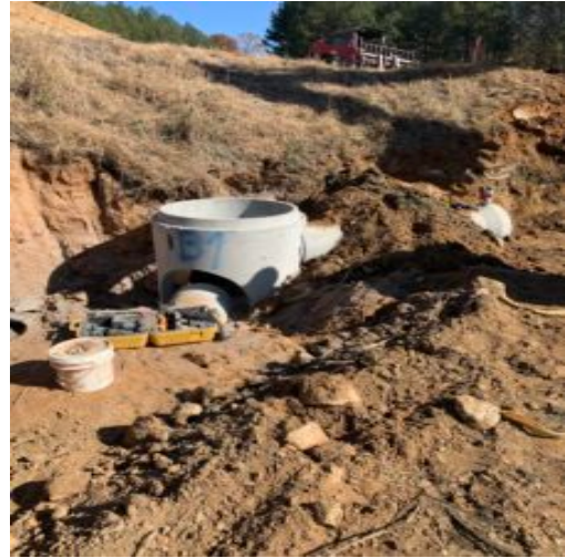
RCP storm installation at bridge embankment
