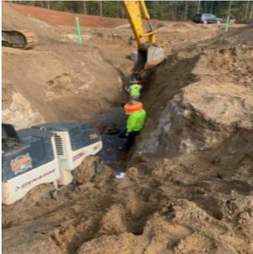
8" d.i.p.sanitary sewer installation between structure #9 and A-9
