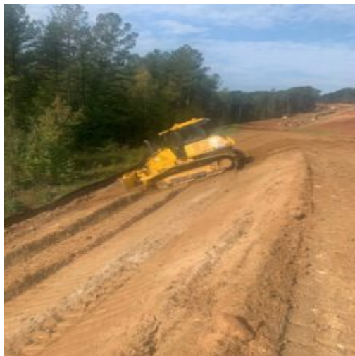
Embankment slope stabilization
