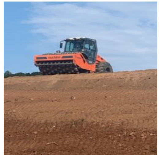
Building lots sub grade compaction
