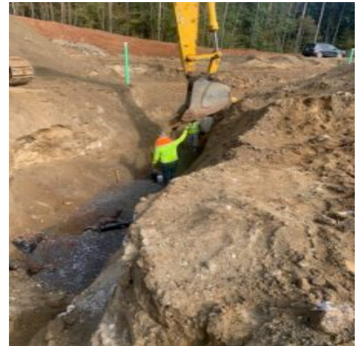
8" d.i.p.sanitary sewer installation between structure #9 and A-9
