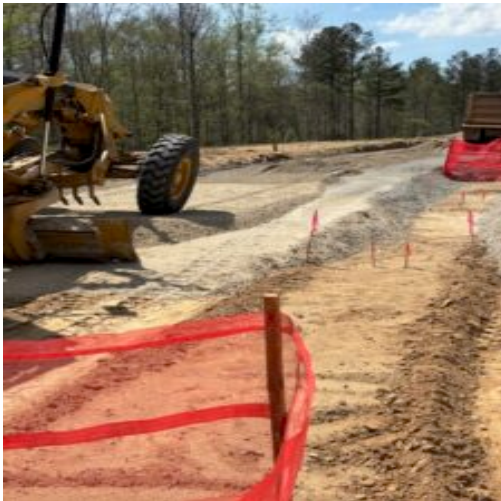
Subbase prep.at Nature Walk Pkwy. between sanitary sewer #4 and6
