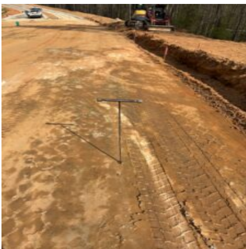
Subgrades observed during proof roll using rounded end steel rod
