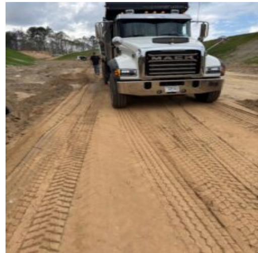
Proof roll observed using loaded tandem dump truck with 18.10 tons
