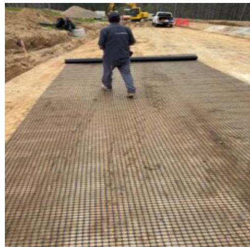
Subgrade prep.installing Tensor stabilization fabric at undercut at Nature Walkway Pkwy. between sanitary sewer manhole # 6 and 4.
