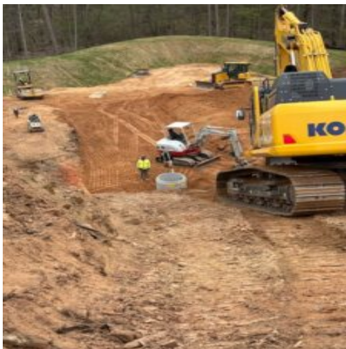
Installation of 36" cmp storm line between A2 and A3
