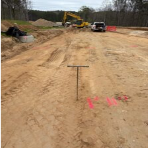
Observe subgrade after undercut
