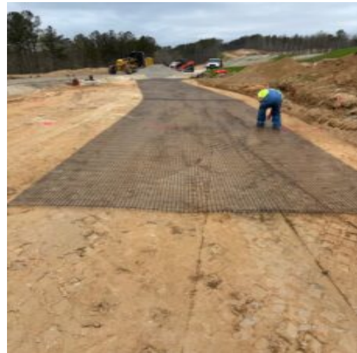
Subgrade prep.installing Tensor stabilization fabric at undercut at Nature Walkway Pkwy. between sanitary sewer manhole # 6 and 4.
