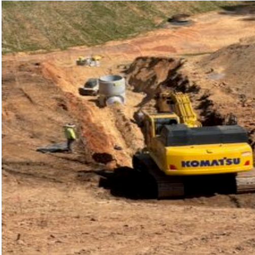
Installation of 30"cmp storm at A line
