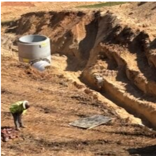
Installation of 30"cmp storm at A line
