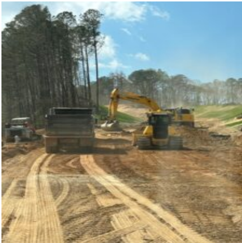
The Grading contractor performing subgrade prep. between
