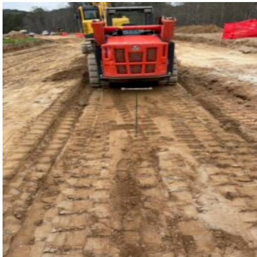
Sub grade prep.at Nature Walk Pkwy. undercut -8"
