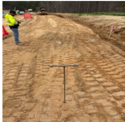
Probing sub grade after undercut
