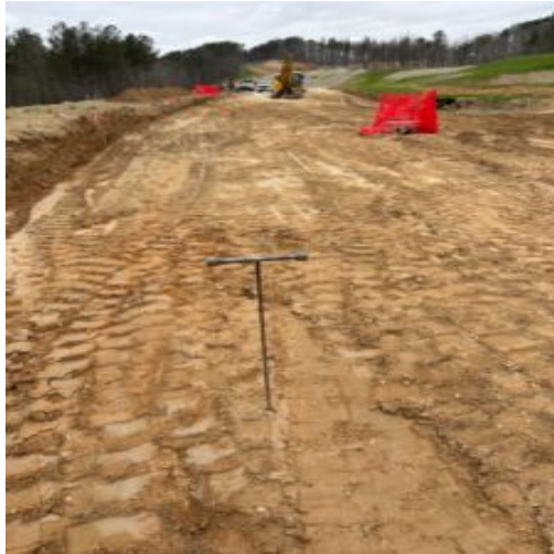
Probing sub grade
