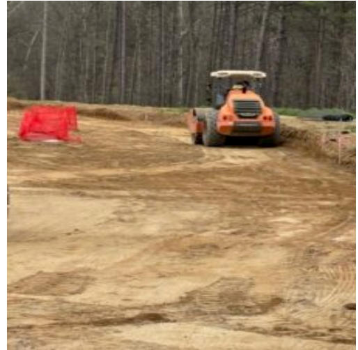
Sub grade prep.compacting using smooth drum roller
