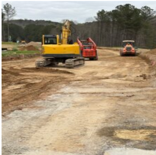
Sub grade undercutting using excavator and skid loader.
