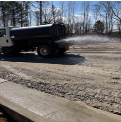
Sub base prep. at Nature Walk pkwy.
