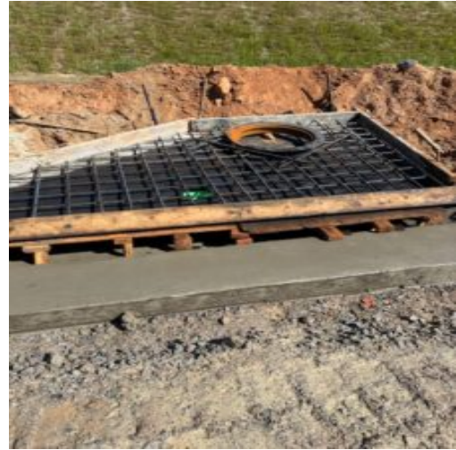
Single wing curb inlet showing reinforcing
