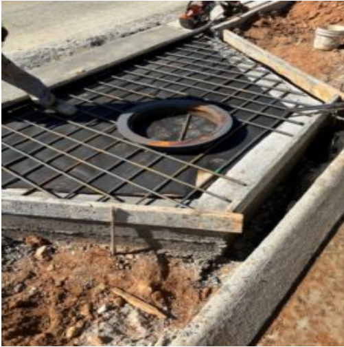
Double wing curb inlet showing reinforcing
