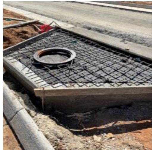
Double wing curb inlet showing reinforcing
