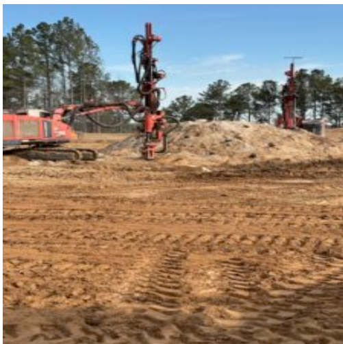
Drilling at lot# 37
