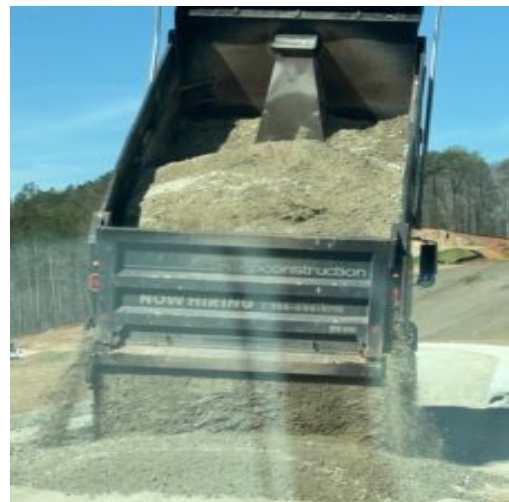
Sub base prep.at Nature Walk pkwy.
