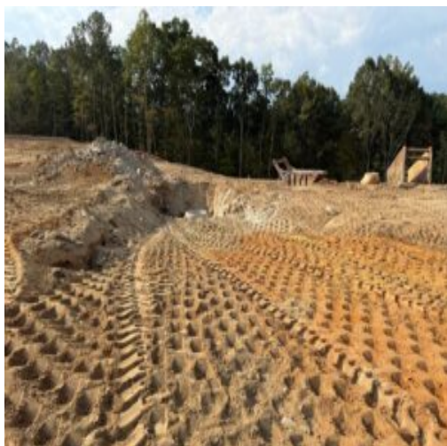
Sewer line backfilling work
