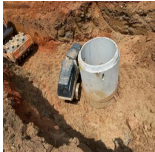
Compaction around the manhole
