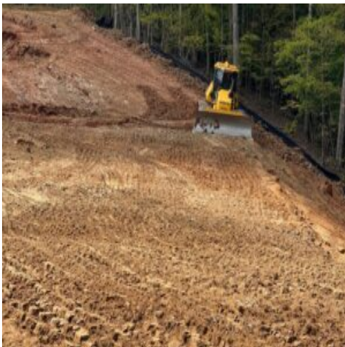
backfilling behind Lot 14 and 15
