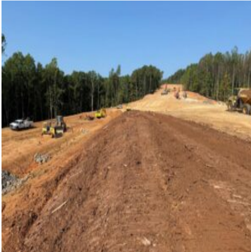
backfilling behind Lot 14 and 15
