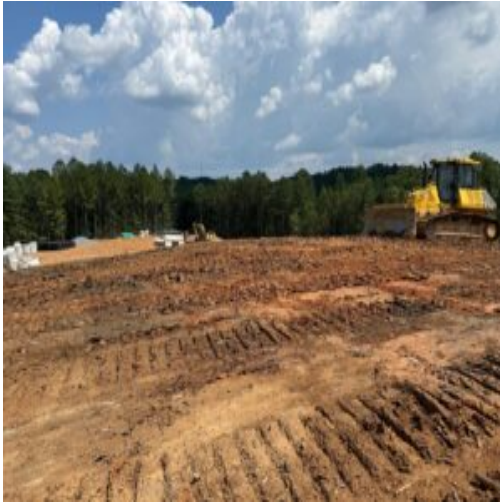
Grading for erosion control
