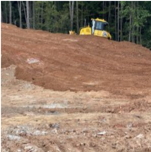
Grading for erosion control
