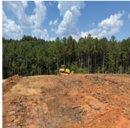
Grading for erosion control
