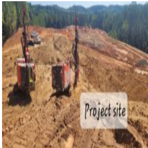
Picture depicting project site with current drilling activities
