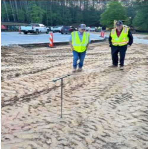
Observing subgrade at east side radius round about to bridge with Thompson Grading and Paulding Co. official using a rounded end steel rod.
