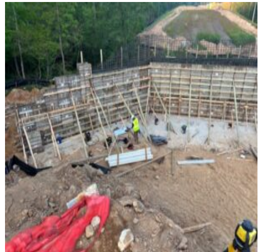
Observing form work prior to concrete pour
