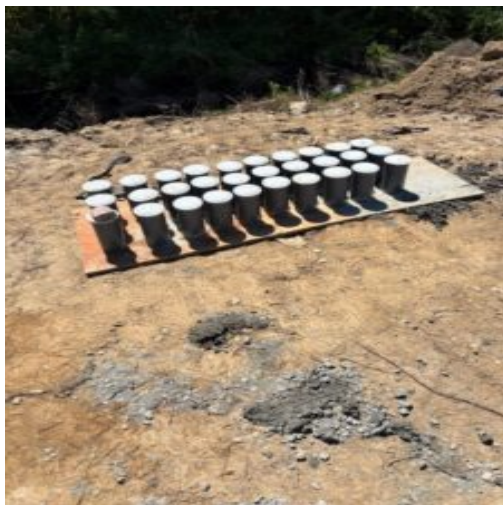
Concrete test cylinders molded
