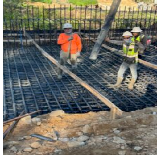
Concrete placement by pumping
