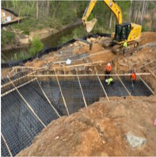
Reinforcing steel in place at Abutment A1
