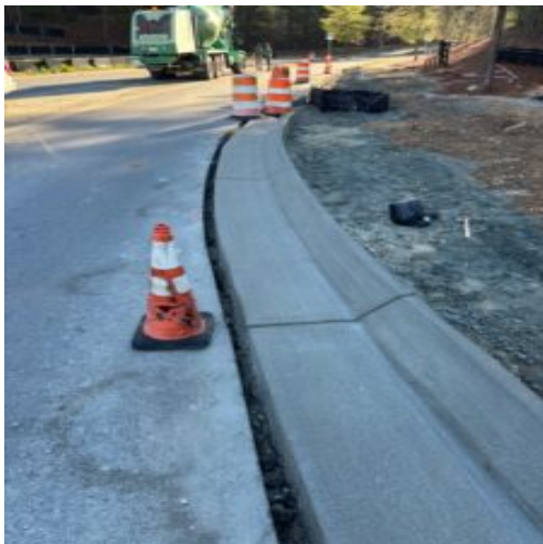
Poured curbing at east side round about
