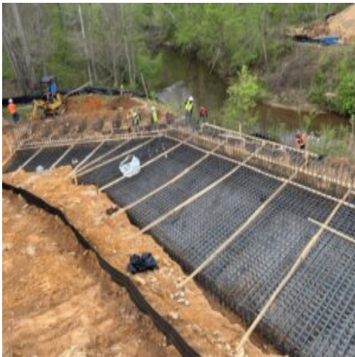
Reinforcing steel in place at Abutment A1
