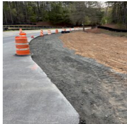
In place sub base stone at east side curbing
