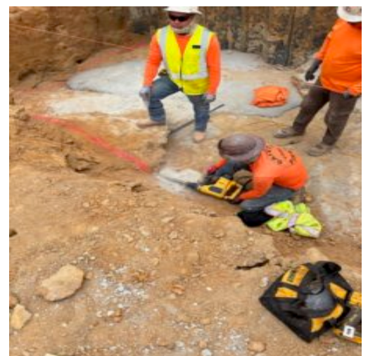
Drilling into existing rock.
