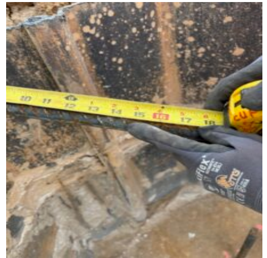
Showing 16" drilled holes.
