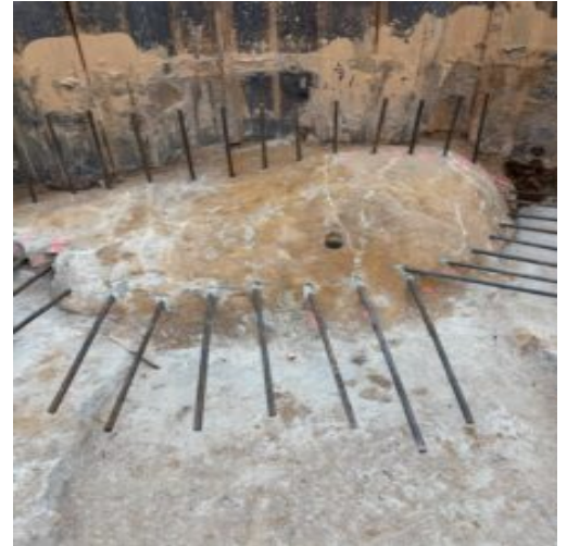
Drilled and epoxied dowels into rock
