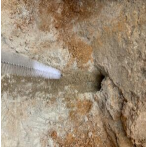
Shows rock dust pulled out of hole
