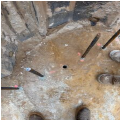
Vertical dowels installed
