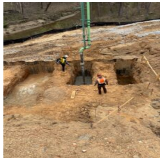
Pouring footings using pump truck
