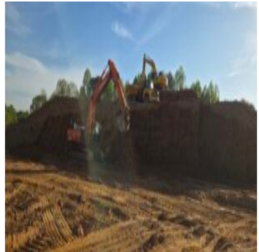
commercial lot excavation
