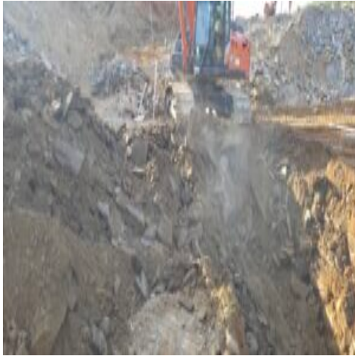
rocky backfill material
