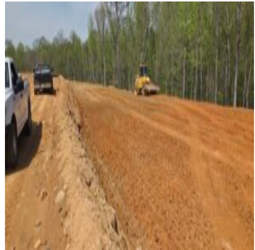
slope on wall 1
