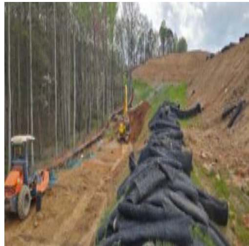
excavation of footing wall 1
