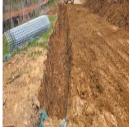
trench for rock in failed area of wall 1
