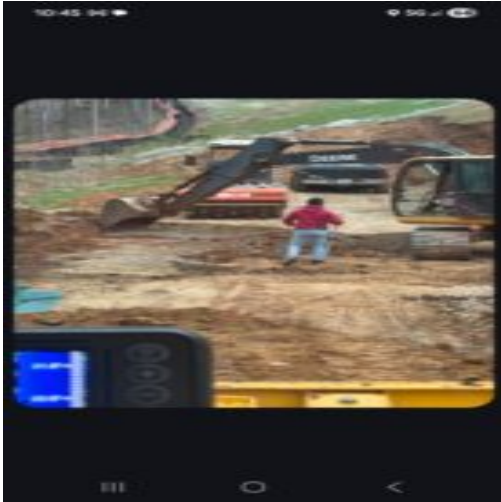
removing the rock in footing wall 1
