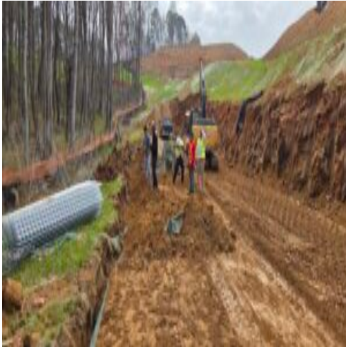
wall 1 contaminated area
