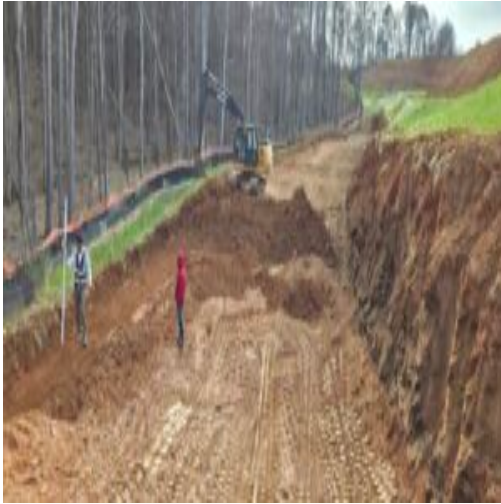
topsoil in footing wall 1
