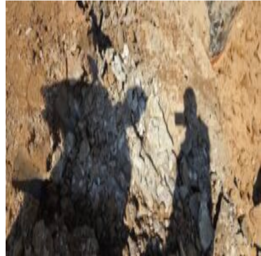
backfill in pipeline area
