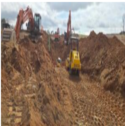
pipeline backfill
