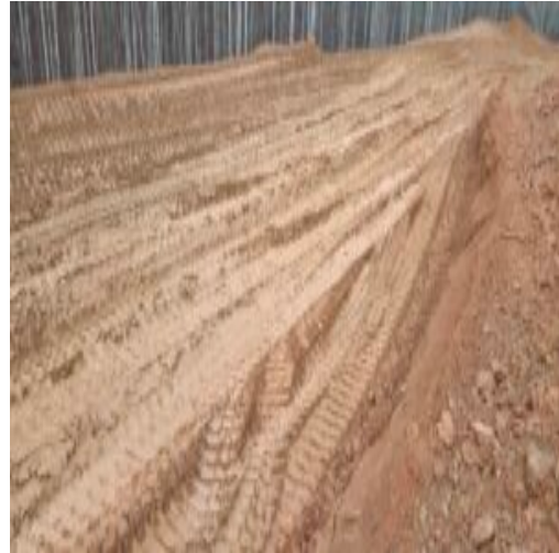
pumping ground by lots 19- 22
