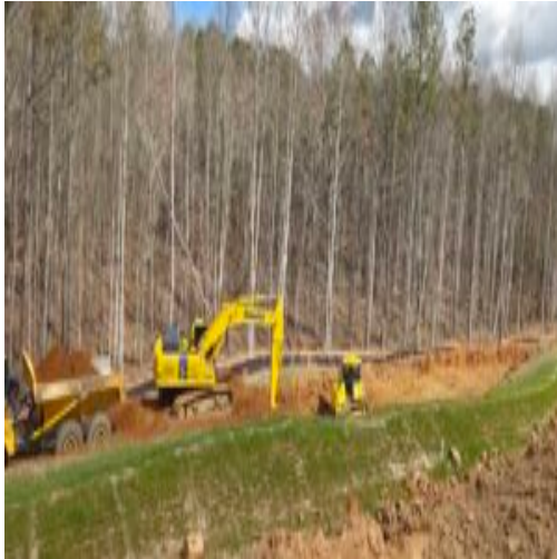
footing wall 1 excavation
