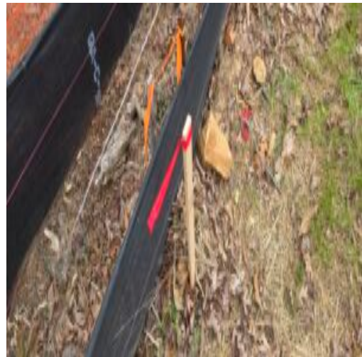
face of wall and lod stakes
