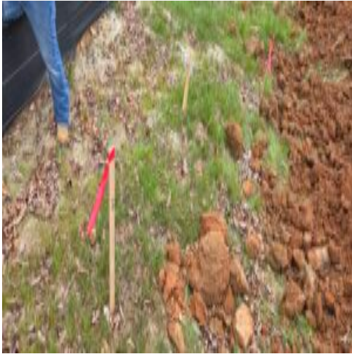
face of wall and lod stakes
