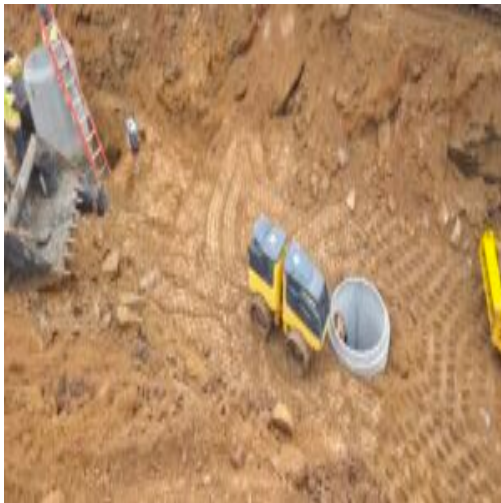
compaction around AA pipeline
