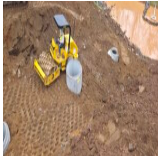
compaction around AA pipeline
