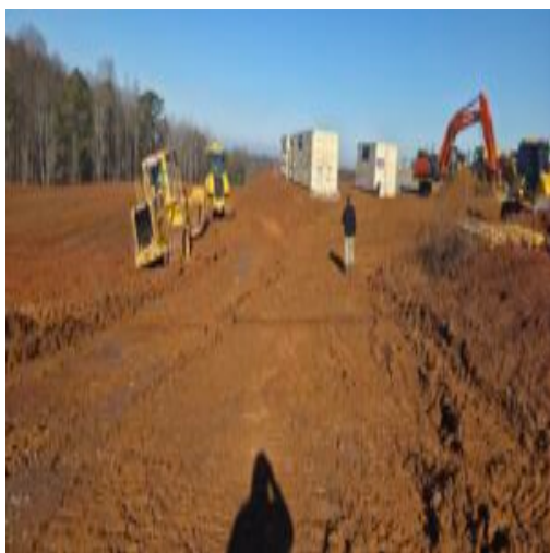
cutting mud/frost out before filling entrance way
