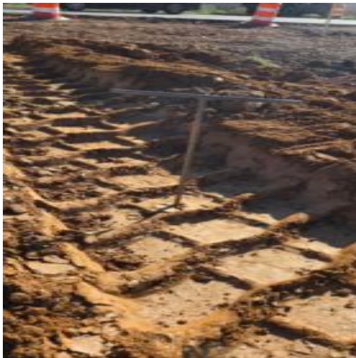
pumping/failed probe rod (addressed by contractor)
