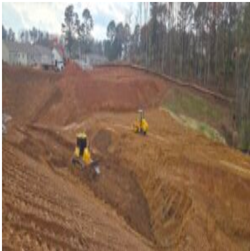
topsoil in bottom of detention pond and filling bank around lot #4 and #5
