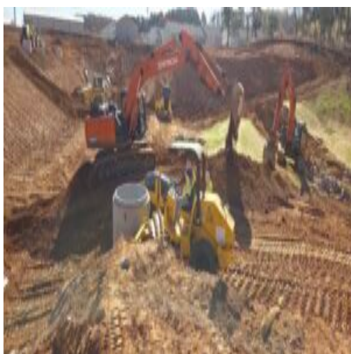
backfilling BZ headwall structure/pipeline
