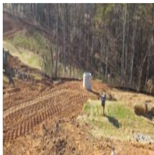
backfilling BZ headwall structure/pipeline
