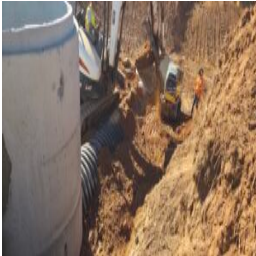
topsoil used as backfill around BA1 to BA2
