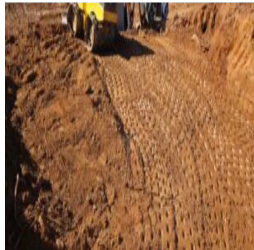
topsoil used as backfill around BA1 to BA2 failing probe rod test
