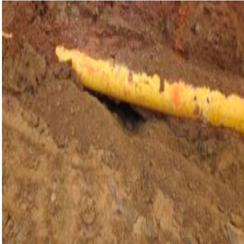
void that was filled under gas line
