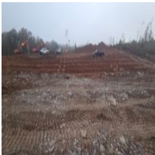
benching into slope for blasted rock fill
