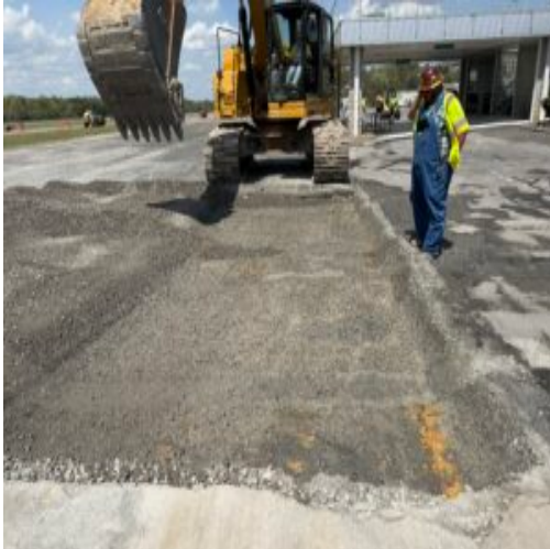
Backfilling with GAB
