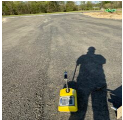
Testing with Gauge
