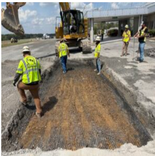
Placing GEO Grid
