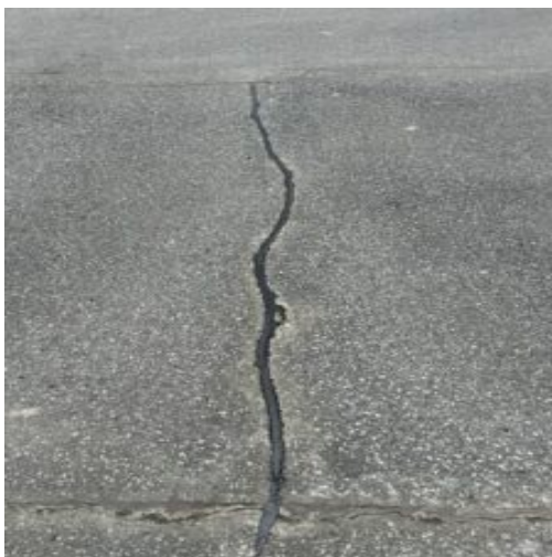
Asphalt cracks cut and filled
