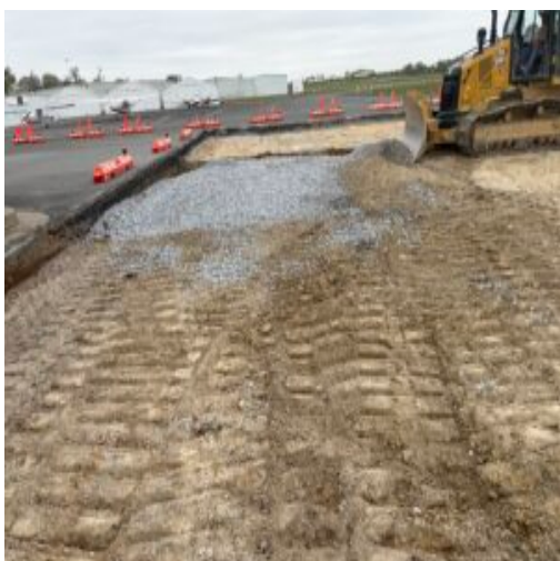
remediation area completed
