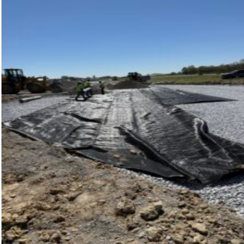
Geofabric placed on #4s
