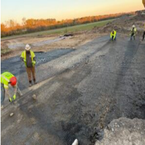
Geogrid placed at corner of A4 and connector.
