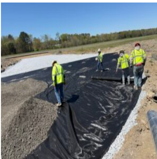
Geofabric placed between #4s and GAB on connector.
