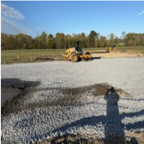
#4s consolidated between A3 and A4 taxiways on connector.
