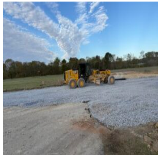
Motor grader for final grade
