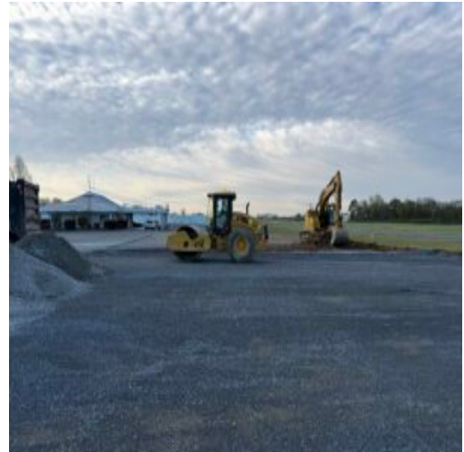
GAB compaction between A3 and A4 taxiways on connector.
