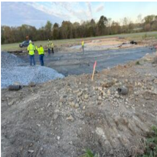
Geogrid placed on subgrade
