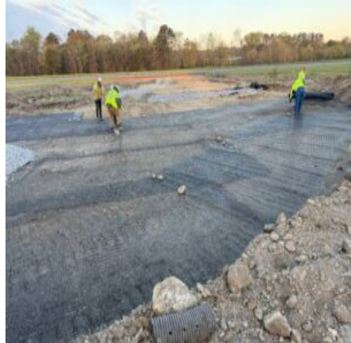
Geogrid placed at A4 and connector.
