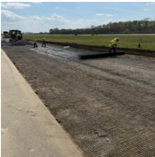
Geogrid being placed between A3 and A4 on connector
