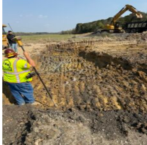
Excavation of pit area.
