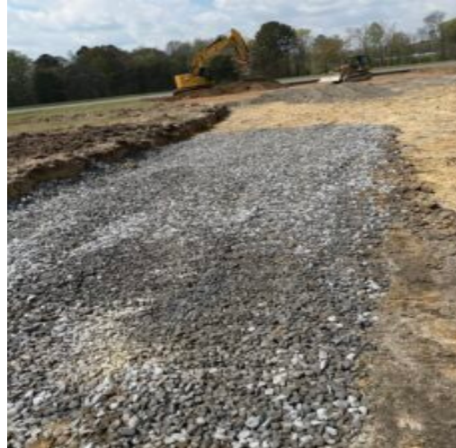
#4s placed on additional remediation area undercut an extra 12 inches below other remediation.
