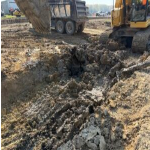
Excavation of Pit area with large organics.
