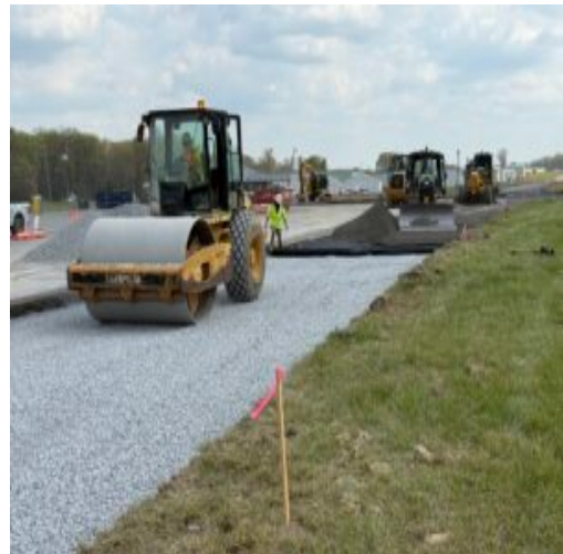
#4s being consolidated on connector between A3 & A4. Picture facing South
