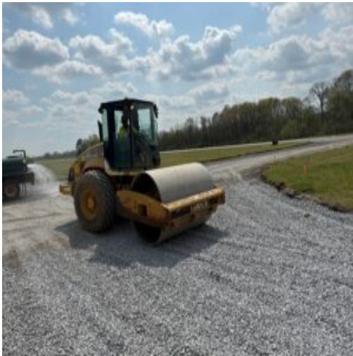
#4s being consolidated at A3 & connector
