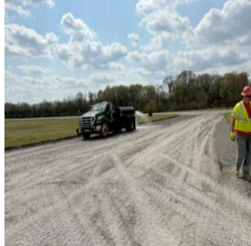
Graded Aggregate Base placed and increasing moisture with water truck.
