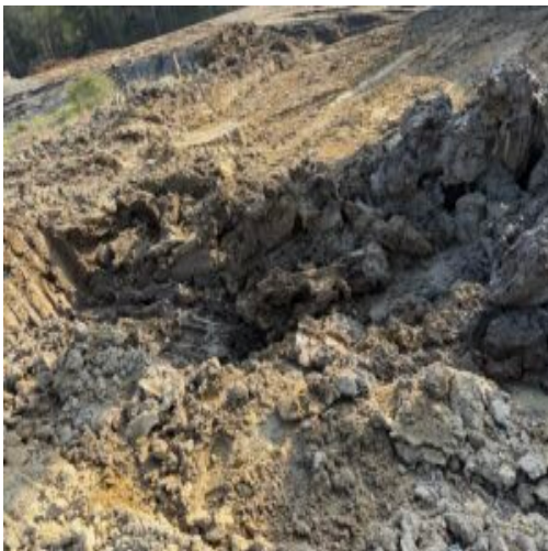
Excavation of pit area with organics
