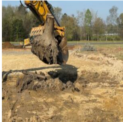
Excavation of pit area (Large tree stump shown being removed)
