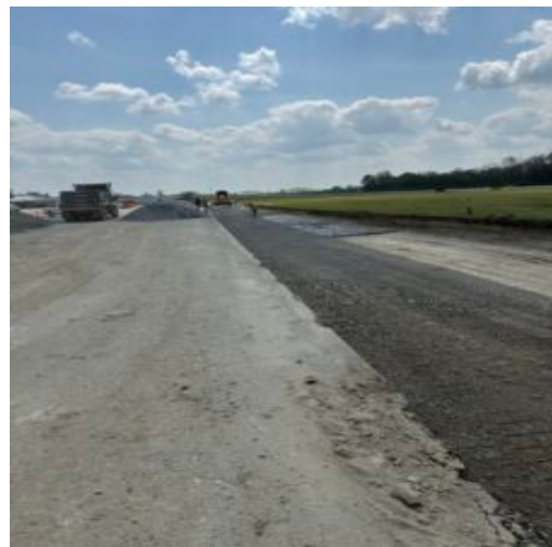
Geogrid bring placed between A3 & A4 on connector
