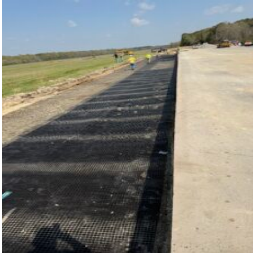
Geogrid placed on connector between A3 &A4. Picture facing North.
