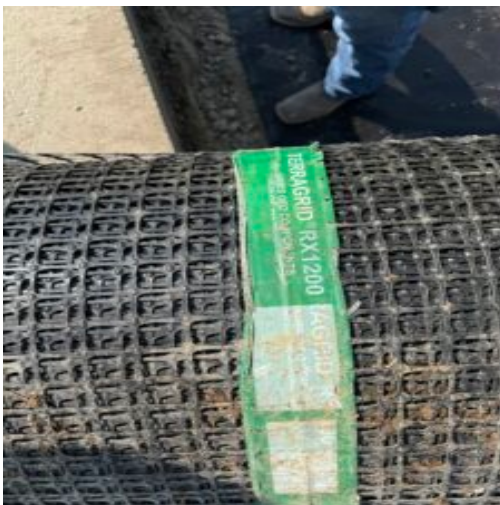
Geogrid being used on this project
