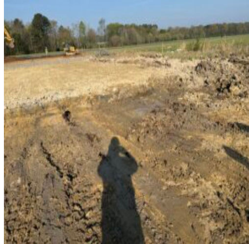
Bury pit area before excavation.
