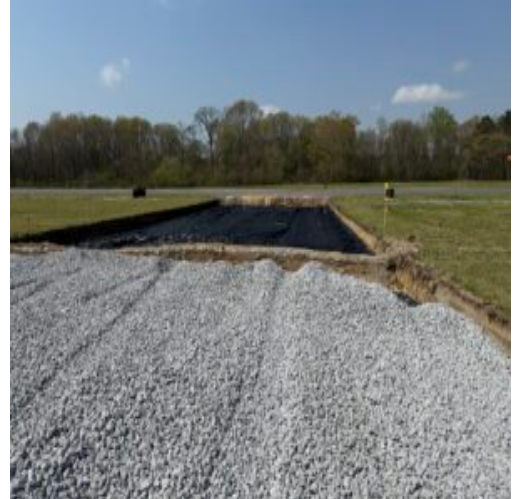
A3 taxiway facing West
