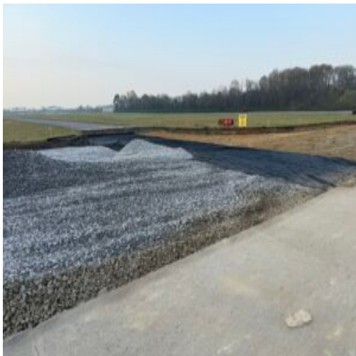
#4 placed on Geo-fabric
