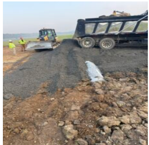
Storm drain material placement A4
