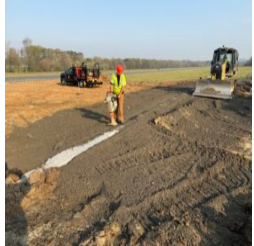
Compacting A4 storm drain sides
