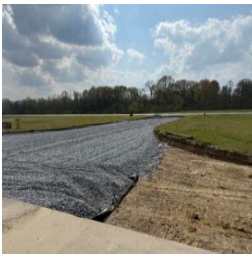
A3 taxiway facing West with #4s placed
