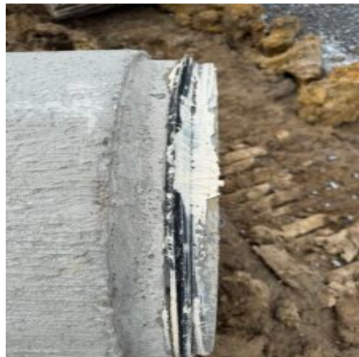
rubber seal and lubricant used on 18 inch RCP
