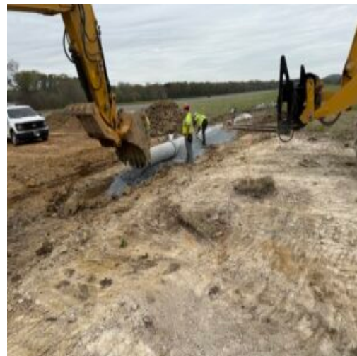
Storm Drain placed
