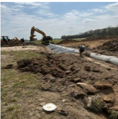
18 inch storm drain facing south
