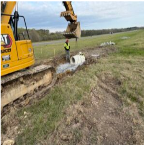
18 inch storm drain placed
