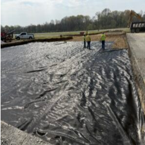
Geo fabric placed
