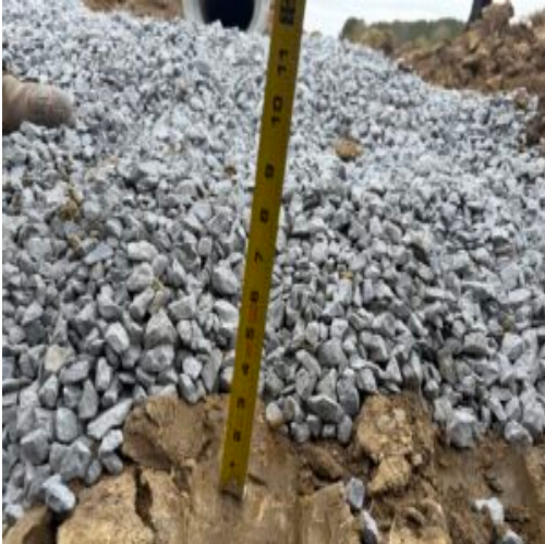
Bedding for Storm drain placed
